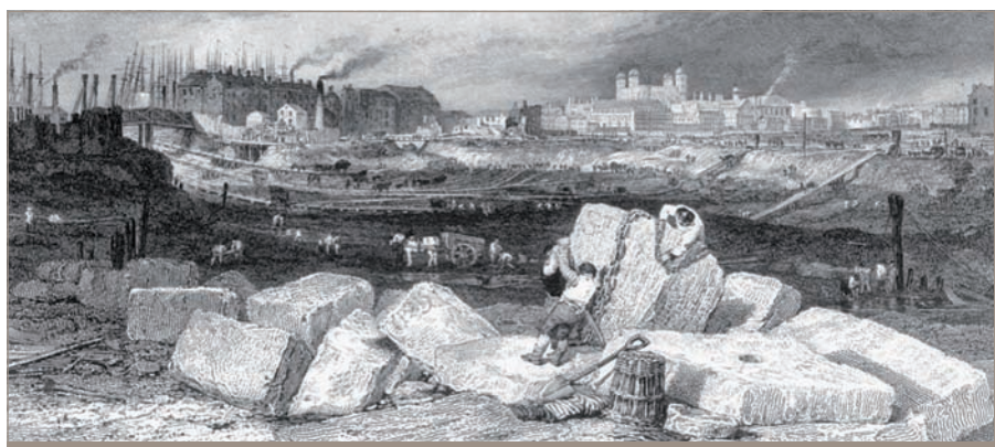
Fig. 5. Excavation in underway in 1827. Spoil was carried in horse-drawn wagons along three iron railways to jetties off the cofferdam, where it was removed by barges (engraving by Clarkson Stanfield)
