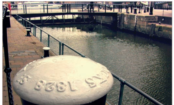
Fig. 12. Telford's entrance lock and all other stone dock structures at St Katharine Docks remain intact today
