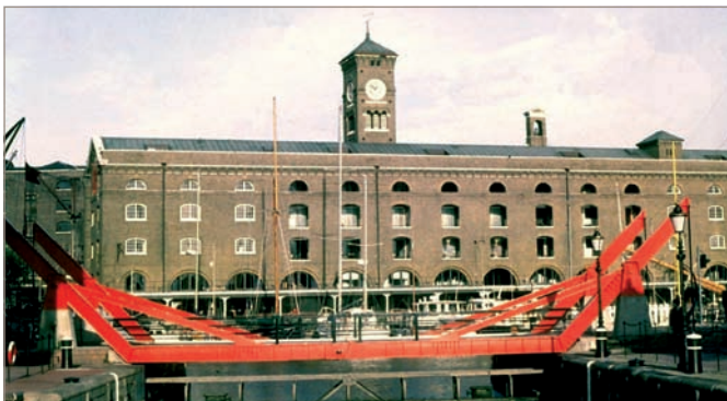
Fig. 11. St Katharine Docks in 1977 following redevelopment as a commercial, residential and marina complex. None of the original warehouses are now left—Ivory House shown here was built in the 1850s (copyright Mike Chrimmes)
